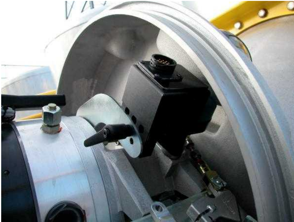
Rotary Transducer on ABB HMB Mech
